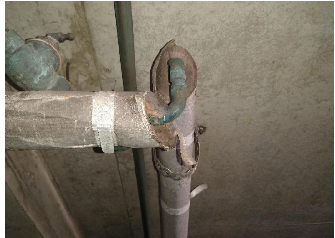
Photo 6: General view of weathered synthetic mineral fibre insulation located in the southern end of the undercroft car park.
