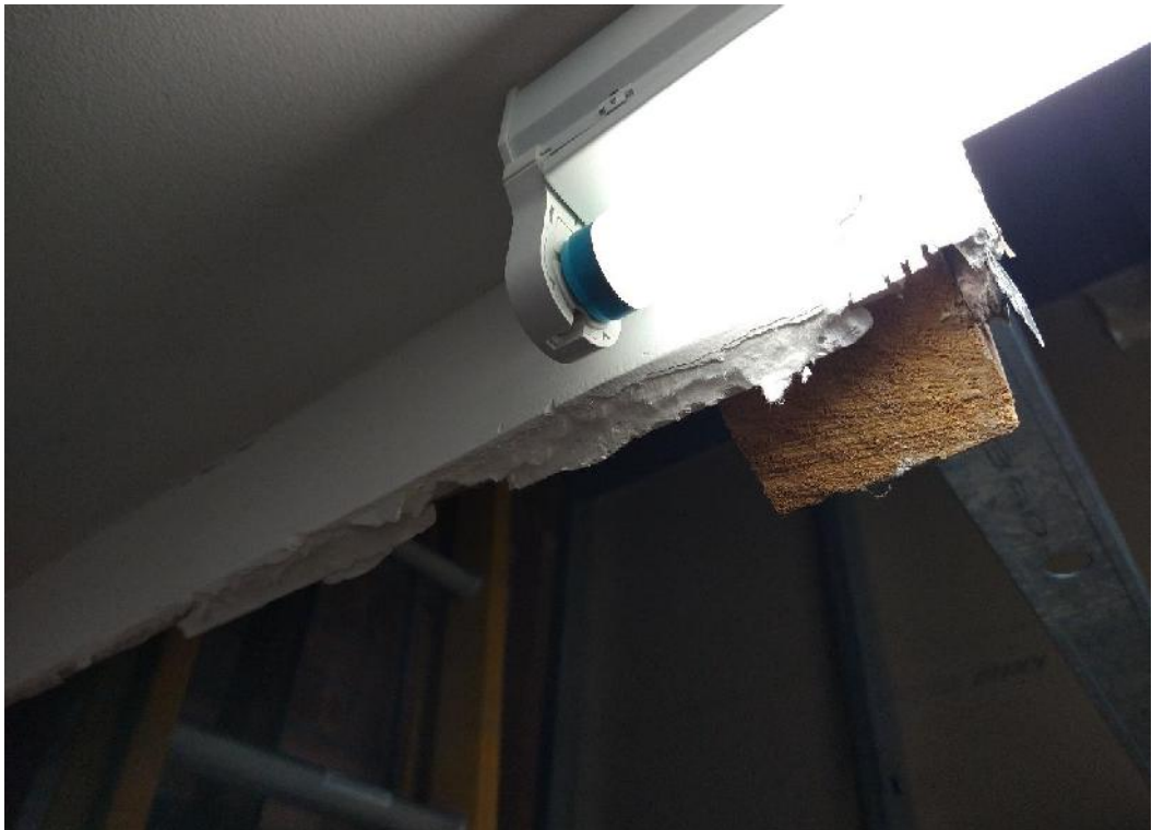
Photo 10: General view of fibrous sheeting located within a storage room located adjacent to the billiards room.
